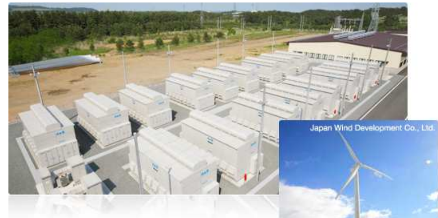
Exemple: 34 MW NAS alongside 51 MW Wind Farm Courtesy of NGK Insulators – Japan)
